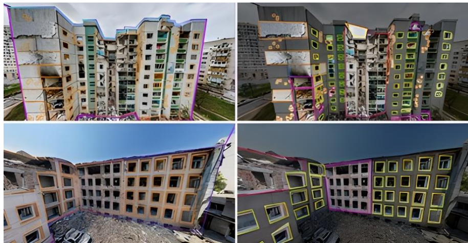
Fig. 10. Comparison of the original and annotated images of damaged buildings
